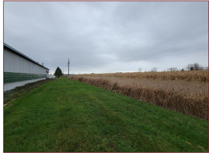
Photograph 2 – Commercial – Light Industry (CVC_2)
