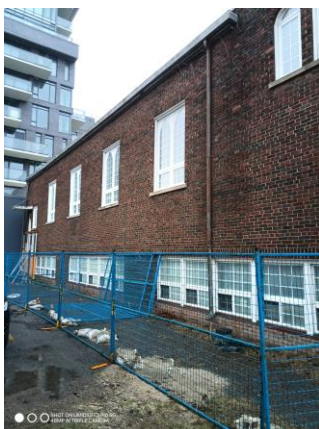
4. Staining of the brick under windows indicates long term water running down the face with cracking from the upper to the lower window.
