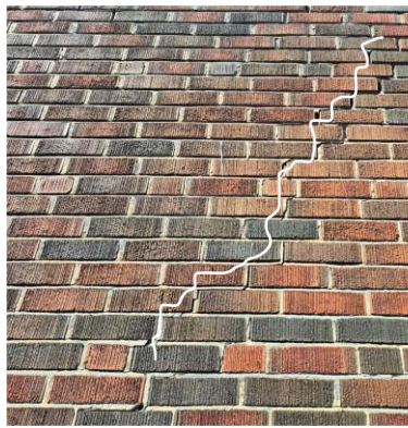
5. Stepped cracks and lost mortar along east façade.
