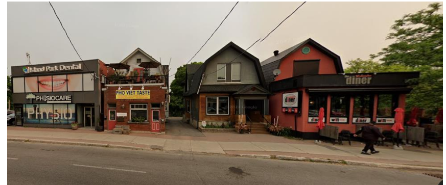
Figure 8 – Existing Buildings to South of Subject Property
