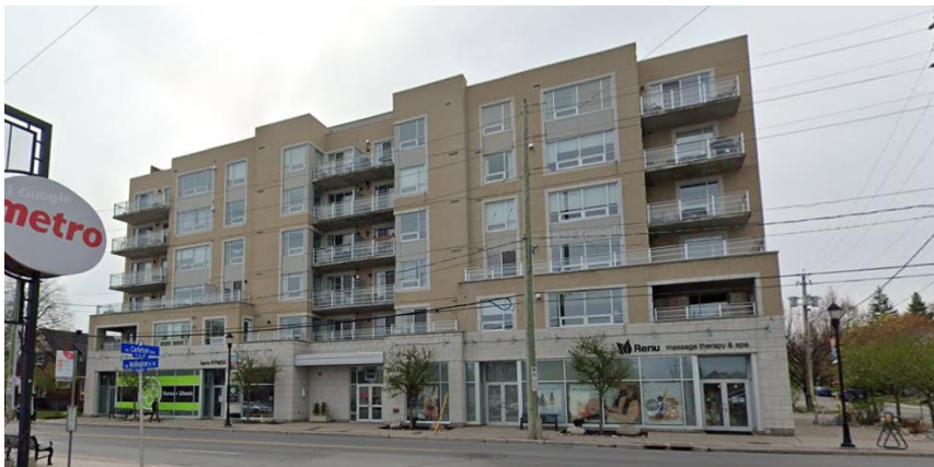
Figure 14 – 6-Storey Mixed-Use Building at 1416-1428 Wellington Street
