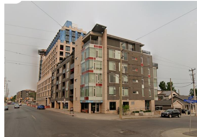
Figure 12 – 6-storey Mixed Use Building at 1433 Wellington Street
