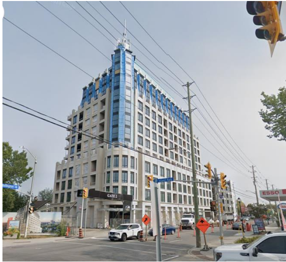
Figure 13 – 11-Storey Mixed-Use Building at 1445 Wellington Street
