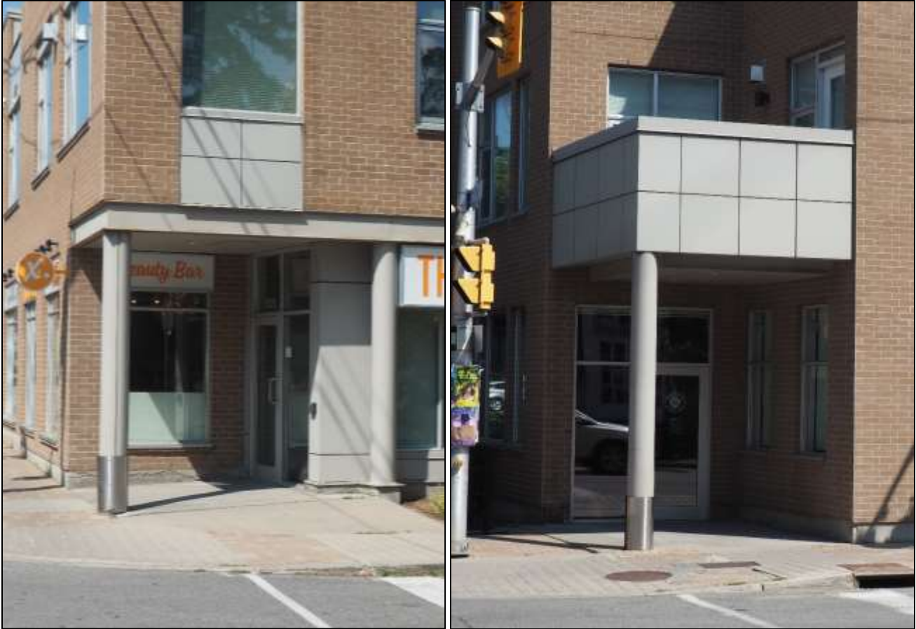
Figure 8: Supported overhangs at the corners of the subject property providing protection from inclement weather for patrons of the uses along the ground floor.
