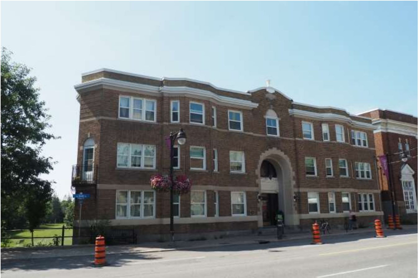
Figure 10: Ambassador Court Apartments as seen from Bank Street looking west.
