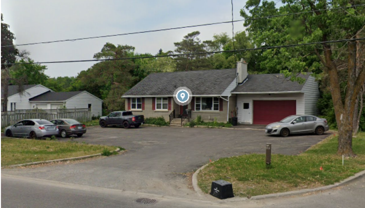
5497 Manotick Main St. Existing building on the subject property
