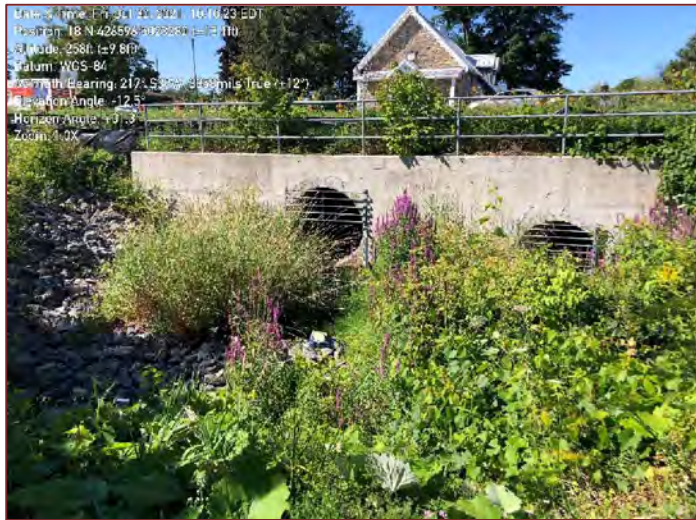
Site Photograph 9 – Inlet for Tributary 4
