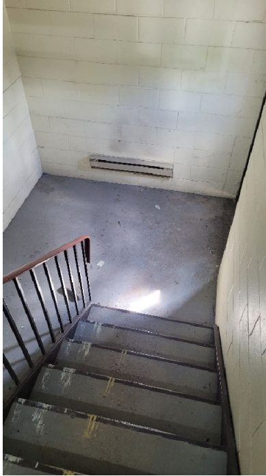
Photograph 7: View of the entry stairwell on the ground floor of the Site building. View also depicts auxiliary baseboard heating.
