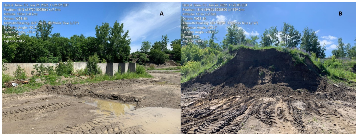
Figure 1 Photographs of the concrete structure in the center of the Site (A) and of a sandbank in the pit (B).
