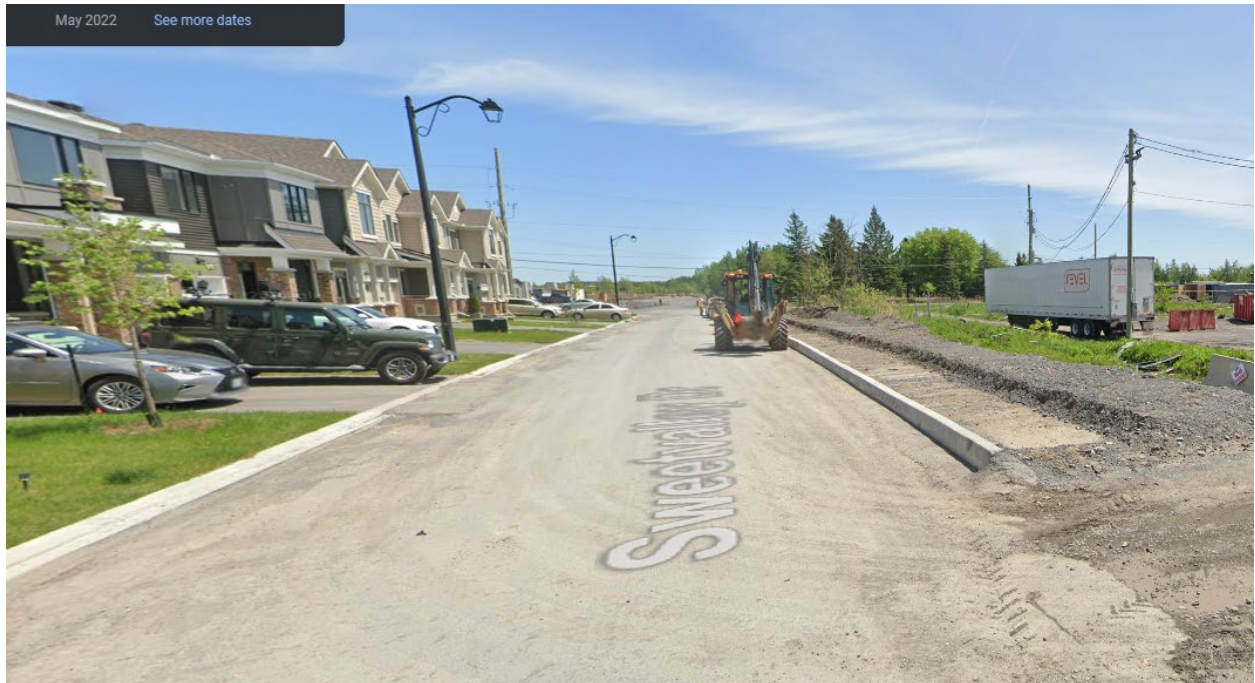
Figure 4: View facing east on Sweetvalley Drive, west of Tenth Line
