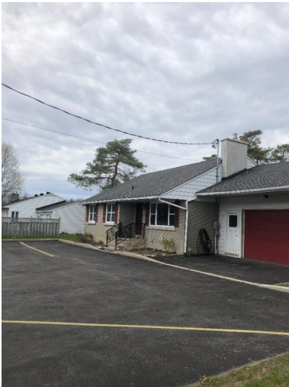
View of front of existing house
