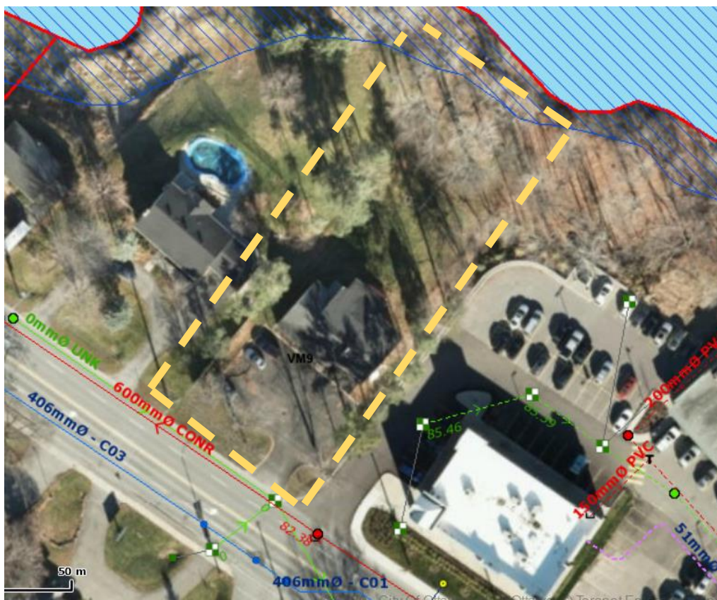
Figure 1- Existing site at 5497 Manotick Main, Manotick, Ontario
