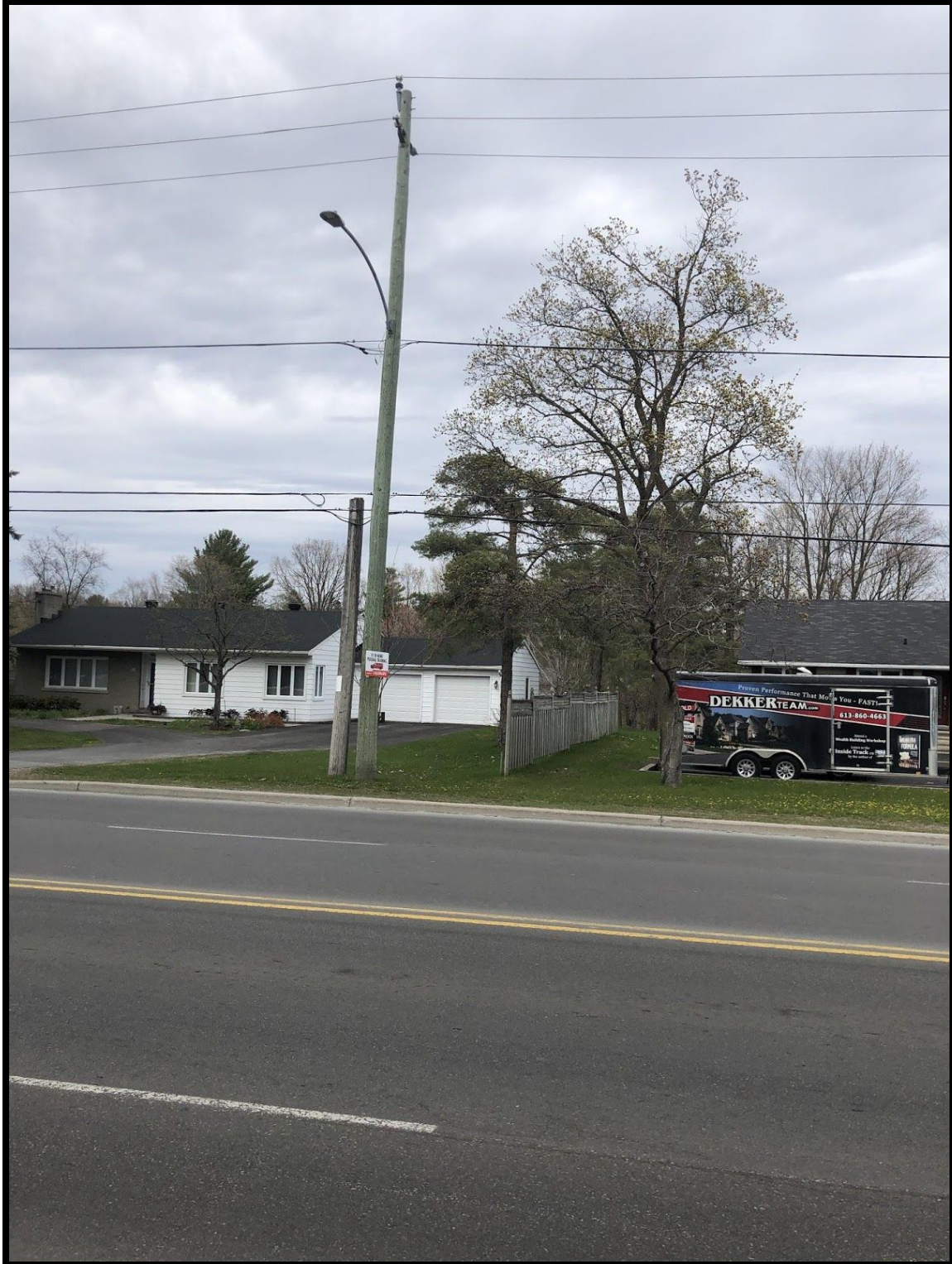
View of the front of the property (north half) taken from Manotick Main Street.
