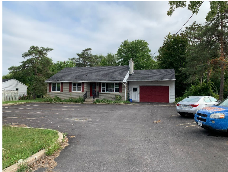
Site Image 02: 5497 Manotick Main Street as seen from street access, with parking at front of site.
