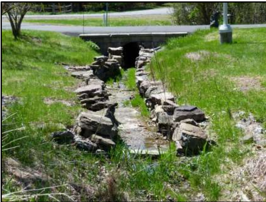
Photograph 19: Upstream (west) section of the Stormwater Swale (Tributary #4). Stormwater flows to the feature from the Marchbrook Circle subdivision and the roadside ditch along Old Carp Road (May 12 th , 2018).
