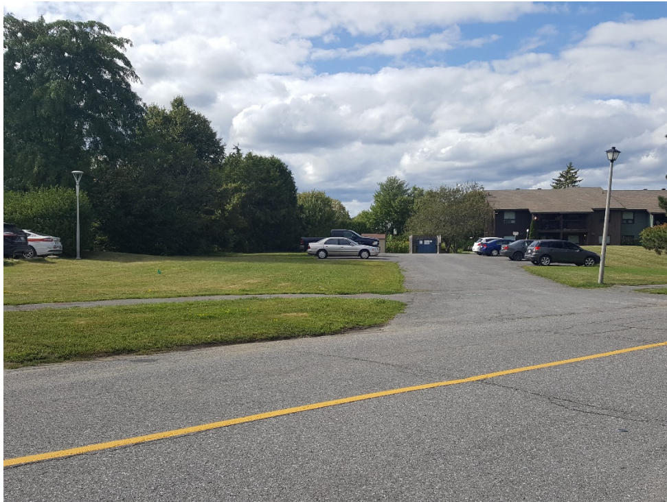
Photo 1 - View of the Site facing north from the south side of Penfield Drive.
