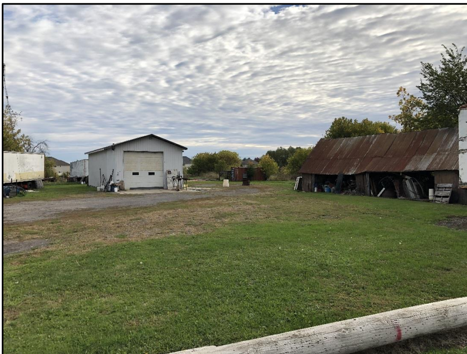
Photograph 2: Southeastern view of the subject site, taken from the west side of the property.
