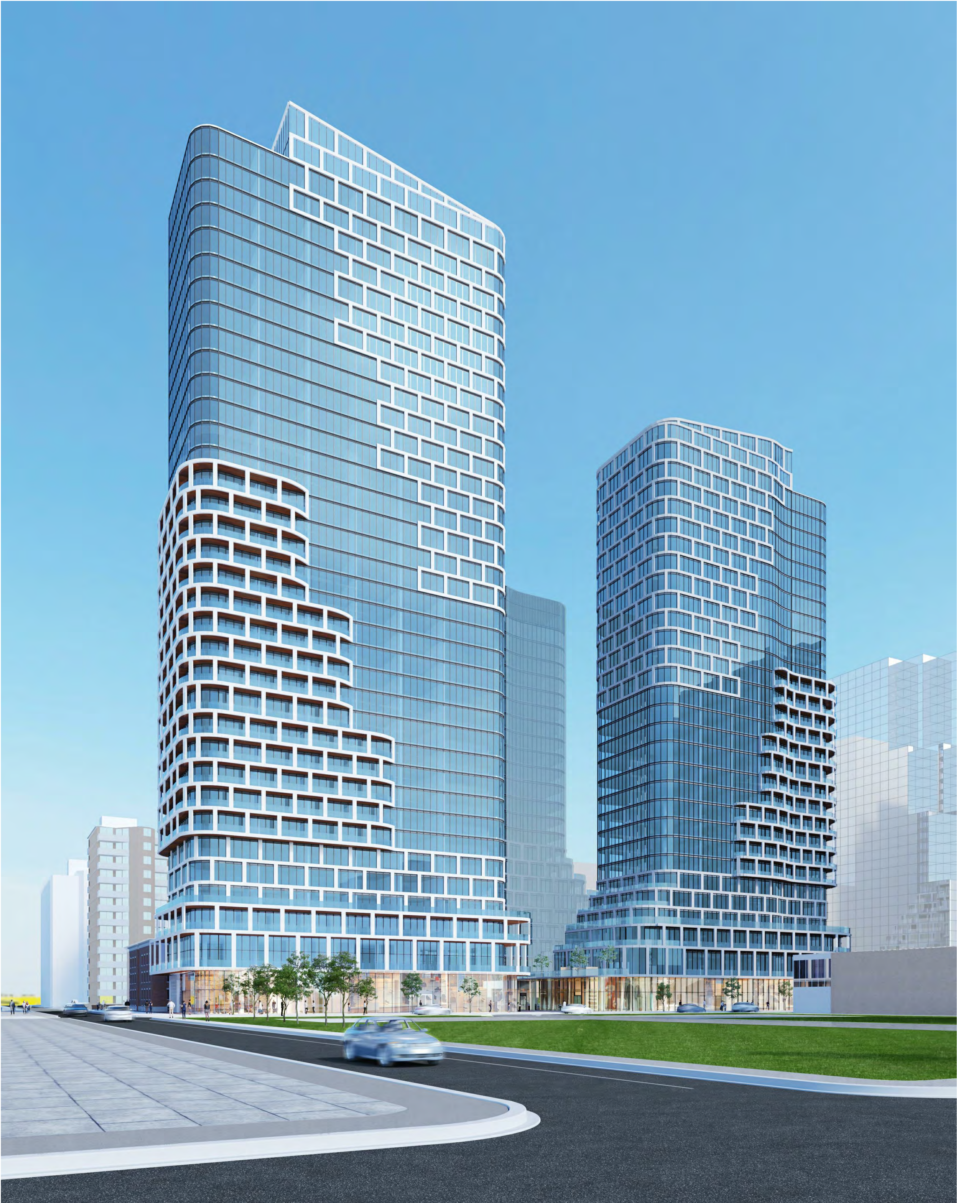
VIEW FROM LYON STREET NORTH LOOKING NORTH
