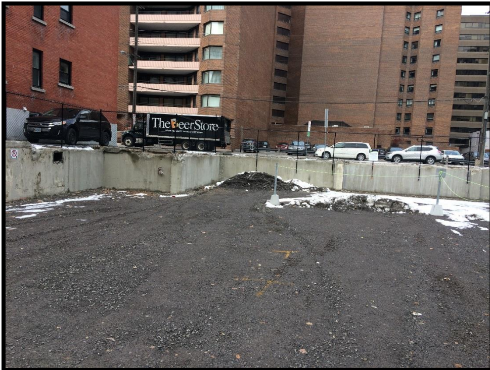
Photograph 4: Retaining walls typical of the northern property line.
