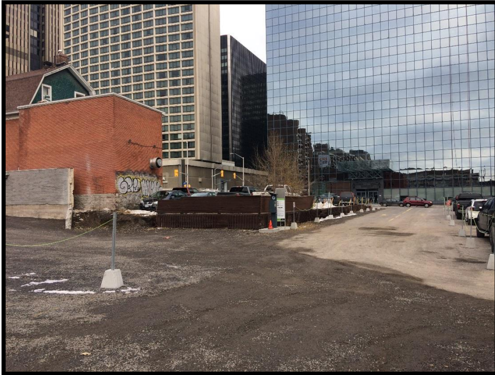
Photograph 1: From the center of the site, looking east. Retaining walls and the two-storey building are visible on the subject site.
