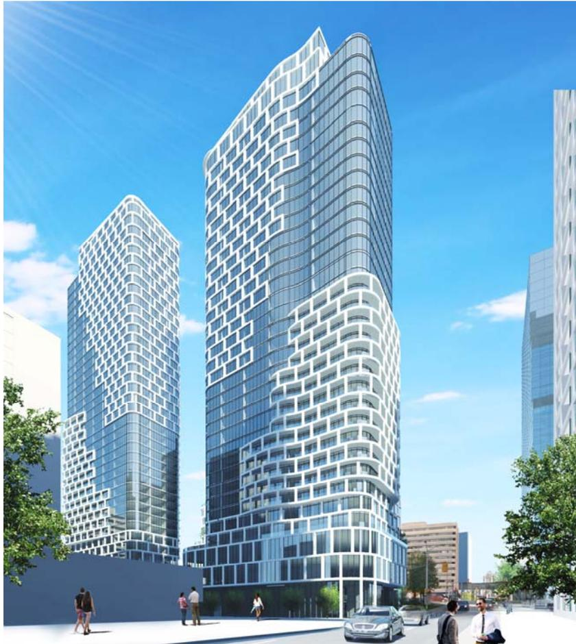
The facades of the 3 towers are composed by a juxtaposition of solid balcony forms framed with a white grid and a glazed tower form.
