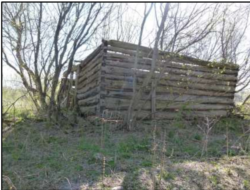
Photograph 47: Building #5 – Looking south at the old barn foundation (May 8 th , 2018).
