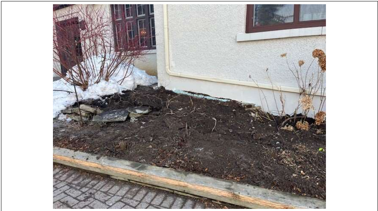
Backfilled pit location
