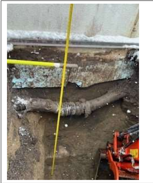
Depth from underside footing to existing grade
