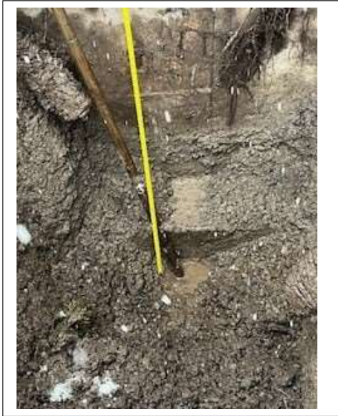
Exposed footing & bedrock surface (ponding water at the bedrock surface)
