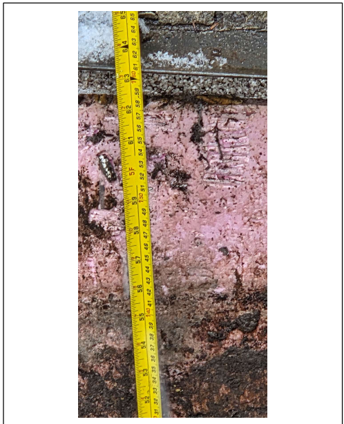
Depth from top of footing to existing grade
