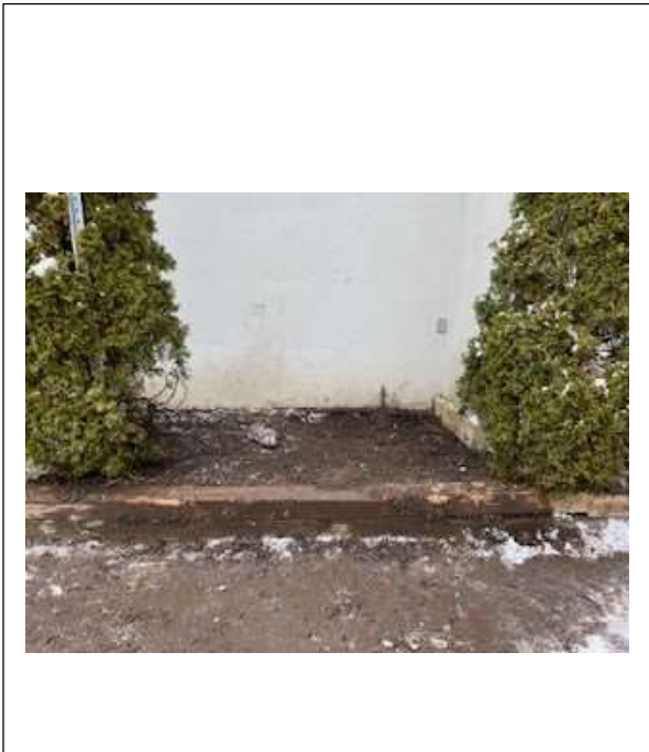
Exposed Bedrock Surface. No Foundation was observed under the adjoining wall
