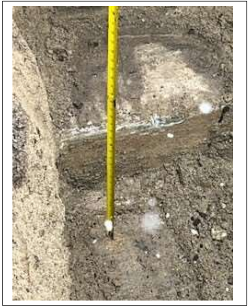
Exposed Footing & Bedrock surface
