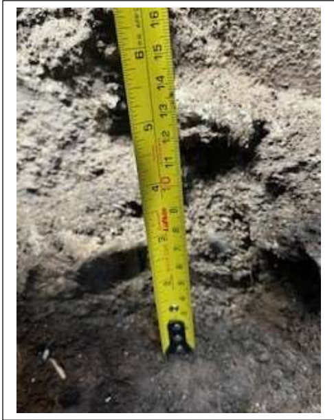
Underside of footing to top of footing (rubble footing)
