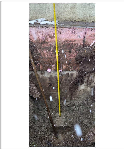
Depth from top of footing to surface
