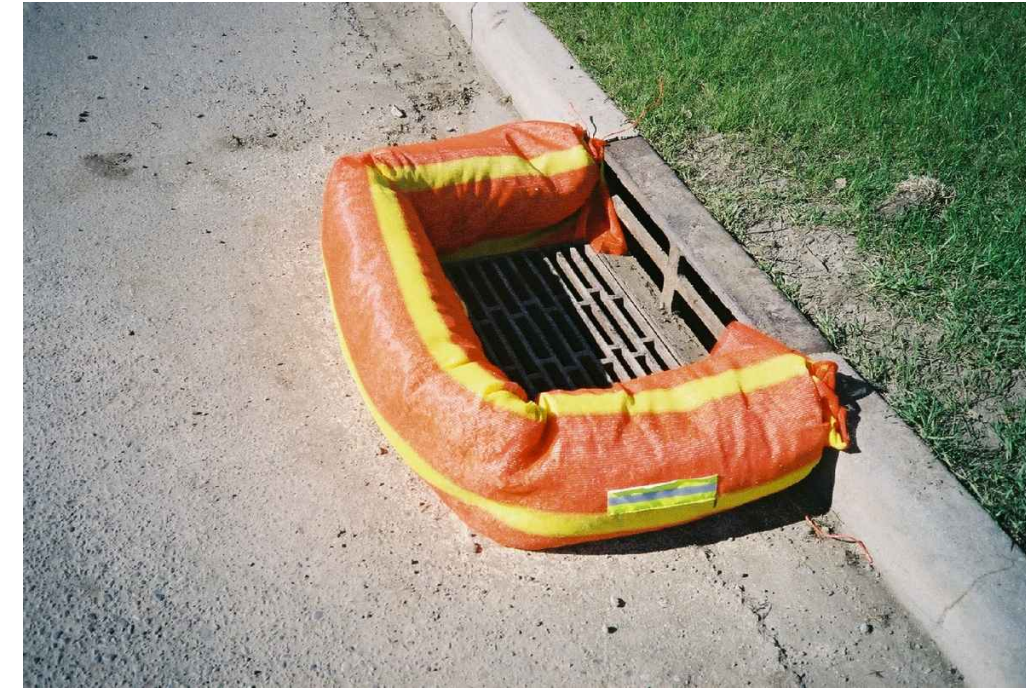
3 TYPICAL SILT CONTROL FOR CATCH BASIN SCALE: N.T.S.
