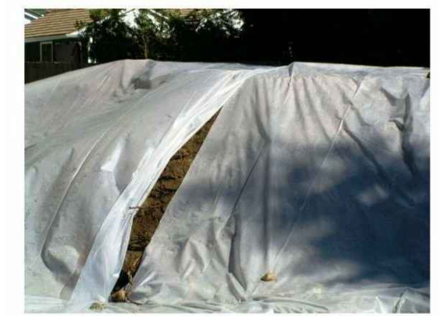
6 TYPICAL SOIL STOCKPILE SCALE: N.T.S.
