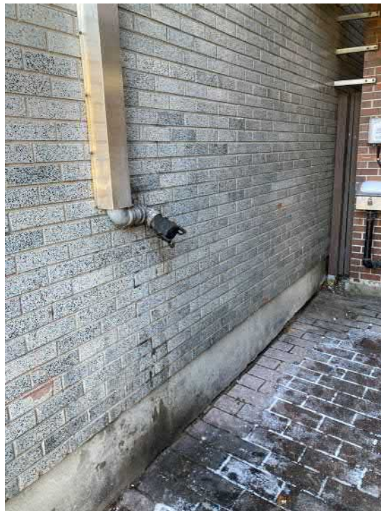
Photo 18: Foreground: grease trap cleanout pipe associated with Clocktower Brew Pub (food grease); vent and fill pipes for diesel generator at adjacent building to north in background
