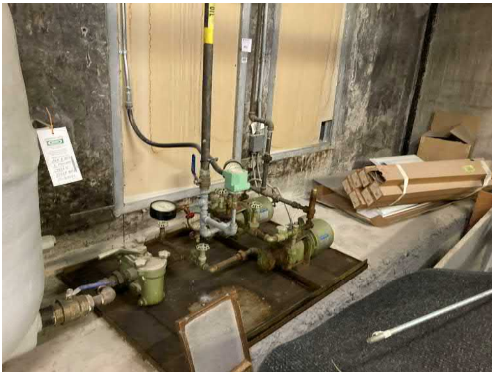
Photo 10: Pumps associated with diesel tank to bring diesel to generator on 11 th floor
