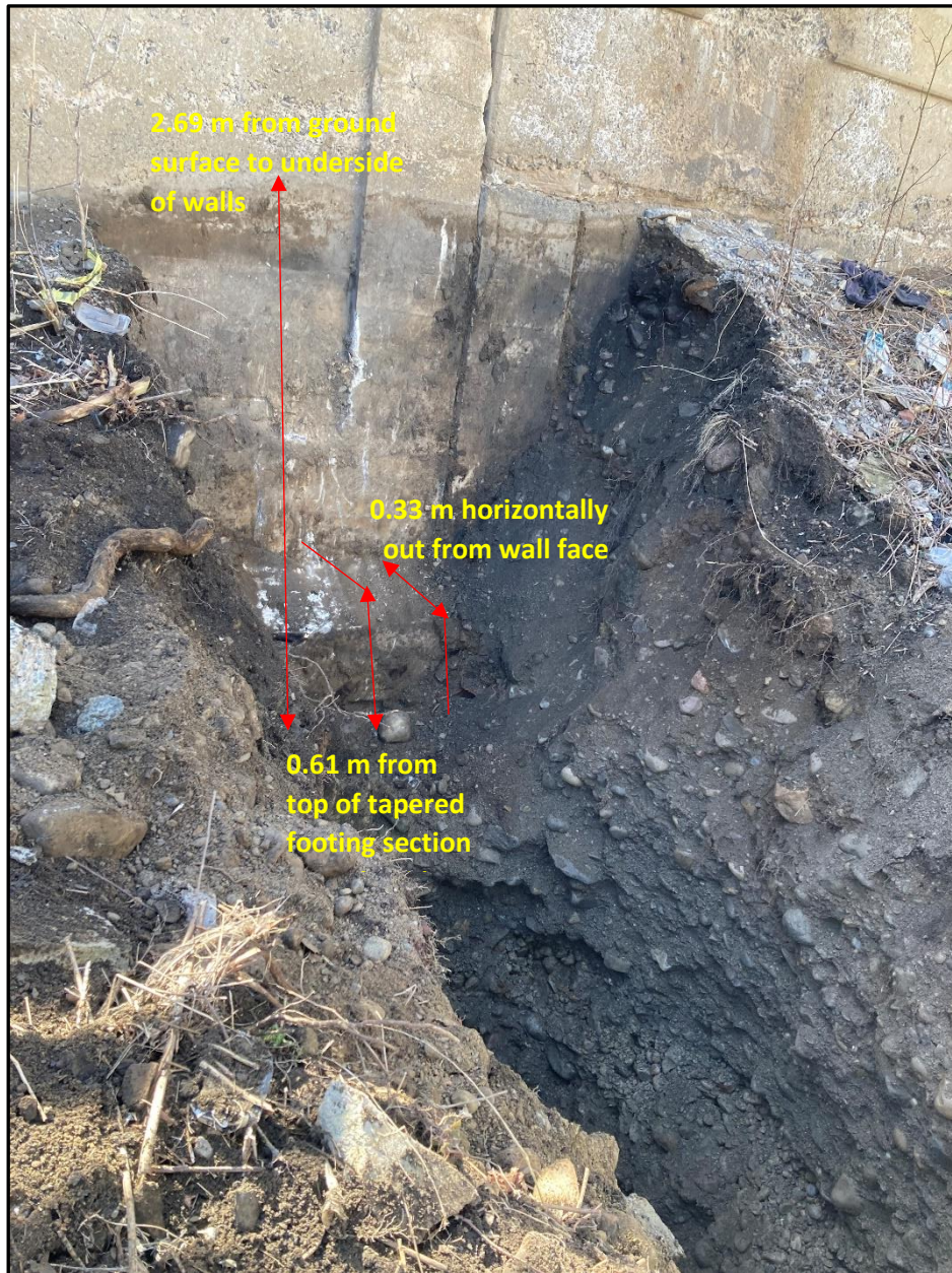
Photo 6 – Details of TP3-22, of the existing retaining wall abutment system for adjacent section of Somerset Street from field program dated April 2022. Wall abutment placed over engineered granular fill.
