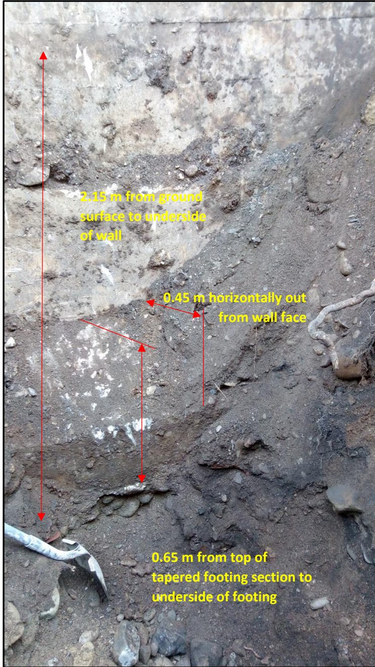
Photo 3 – Details of existing retaining wall abutment system for adjacent section of Somerset Street from field program dated December 2019. Wall abutment placed over engineered granular fill.
