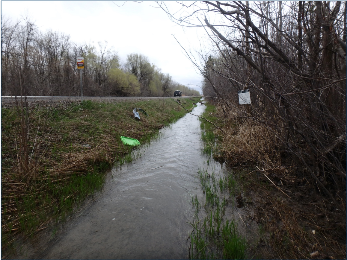
Photo 3: Photo showing roadside ditch along Rideau Road during freshet flow conditions northwest of the subject property. Photo facing northeast (Photo Date: April 16th, 2021).
