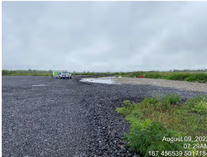
Photo 1 - View of drilled water well on the Site used during pumping test and proposed building area showing ground improvement.
