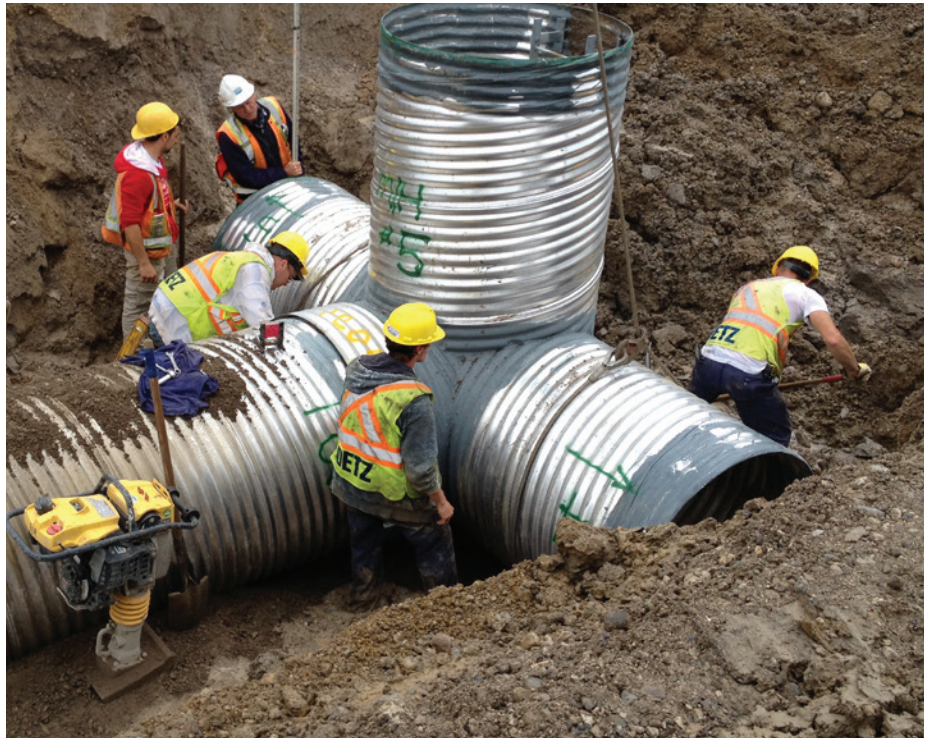
STEELCOR'S LIGHTWEIGHT SECTIONS ALLOW INSTALLATION WITHOUT THE NEED FOR HEAVY EQUIPMENT
