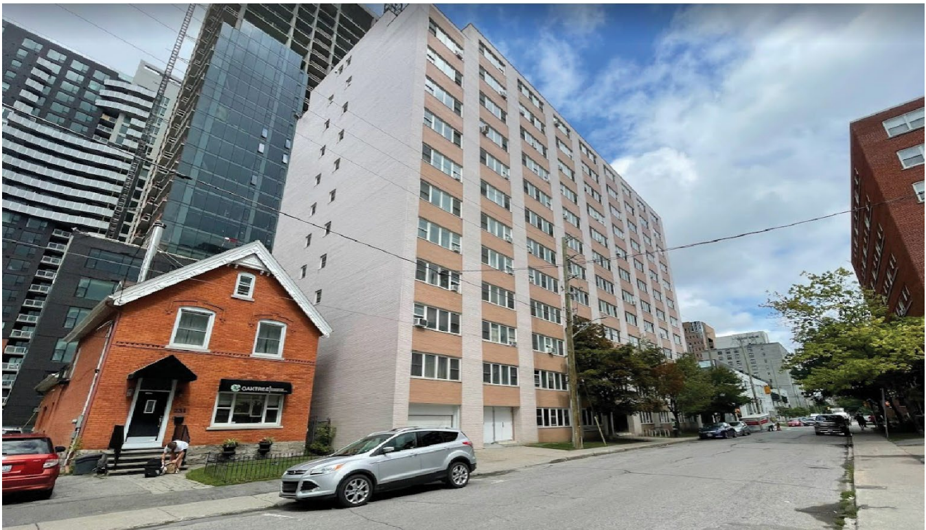
Figure 2: Site context, looking north
