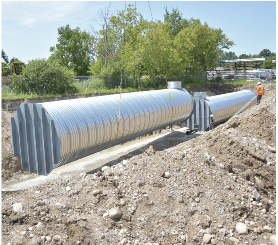
HELICAL CORRUGATIONS AND CONTINUOUS LOCK-SEAM PROVIDE STRENGTH IN A LIGHTWEIGHT STRUCTURE
