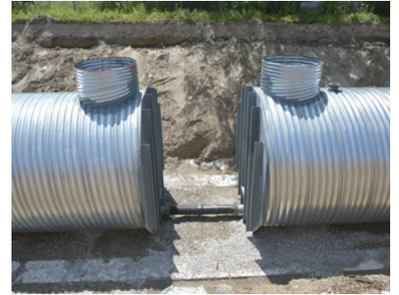
GALVANIZED CSP FIREWATER TANK SYSTEM
