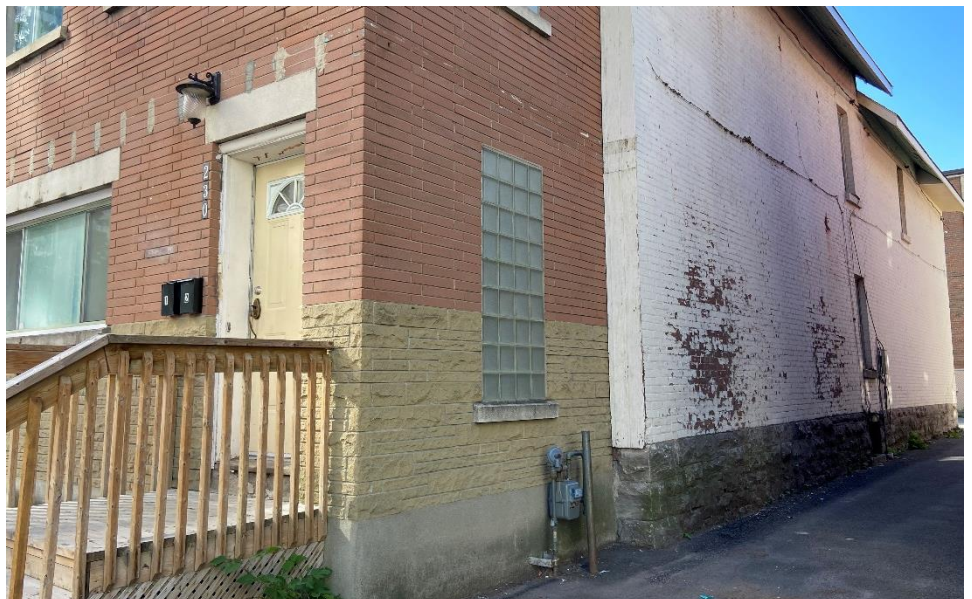
7 Close up of brick addition to the front of 230 Lisgar showing the connection between old and new. MTBA
