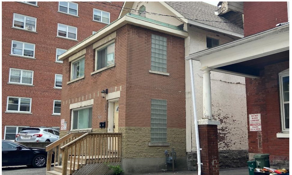
6 Brick addition to the front of 230 Lisgar. MTBA
