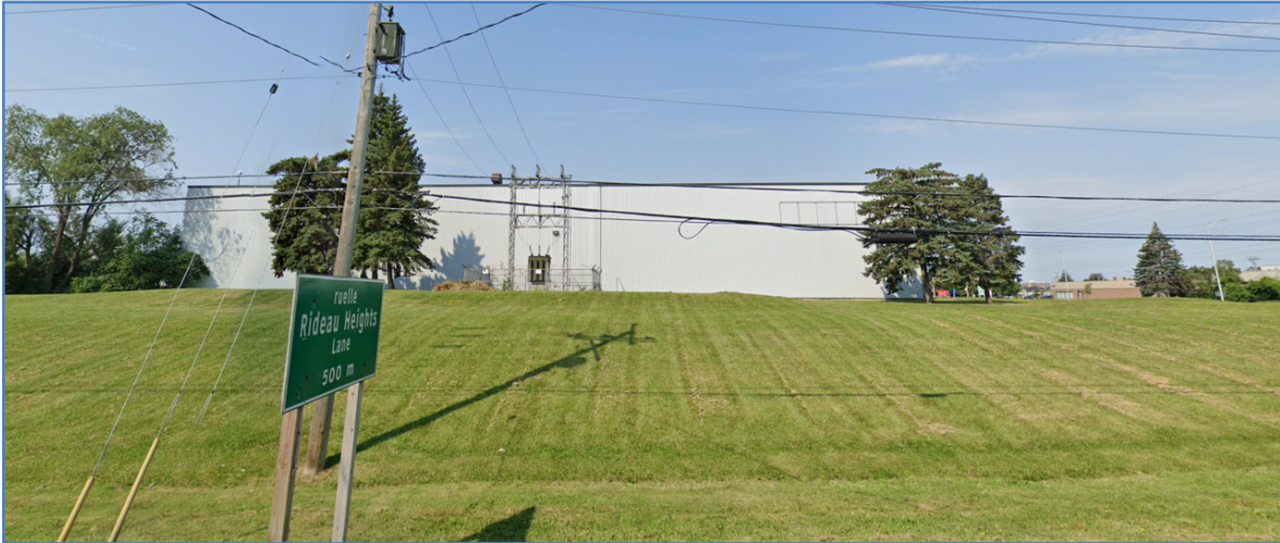
Existing Site Conditions: Facing West
