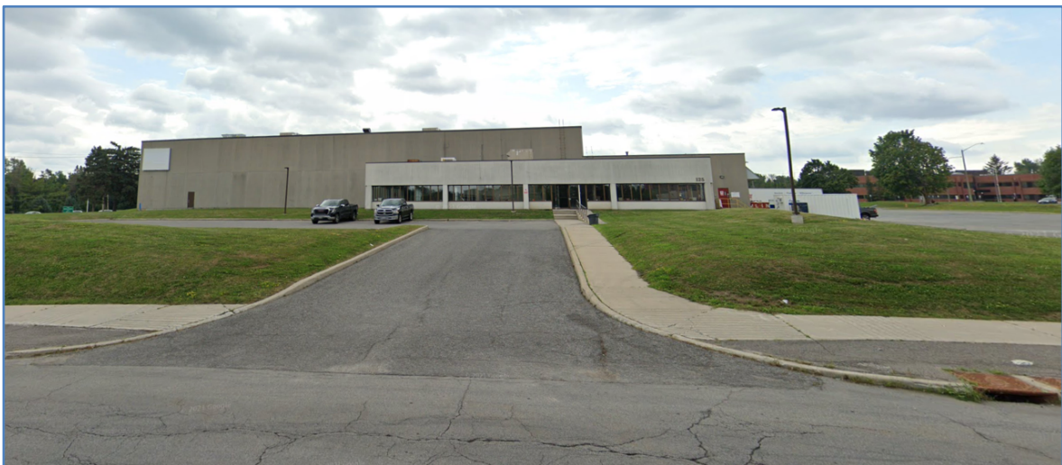
Existing Site Conditions: Facing South
