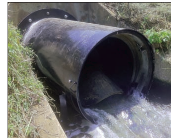
CheckMate® Thimble Insert
