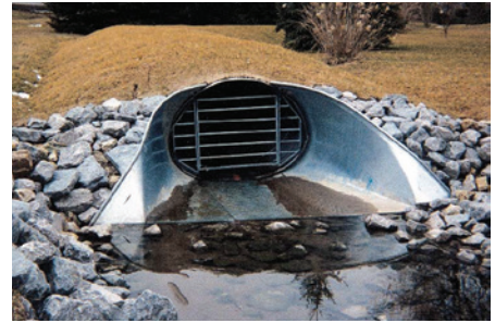
CSP END SECTION WITH FUNCTIONAL GRATE
