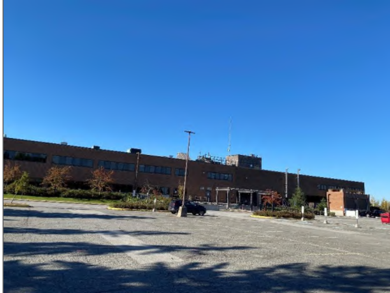
Photo 9 – Electronic and computer equipment manufacturer located adjacent to the southwest elevation of the Phase One Property (PCA #1).
