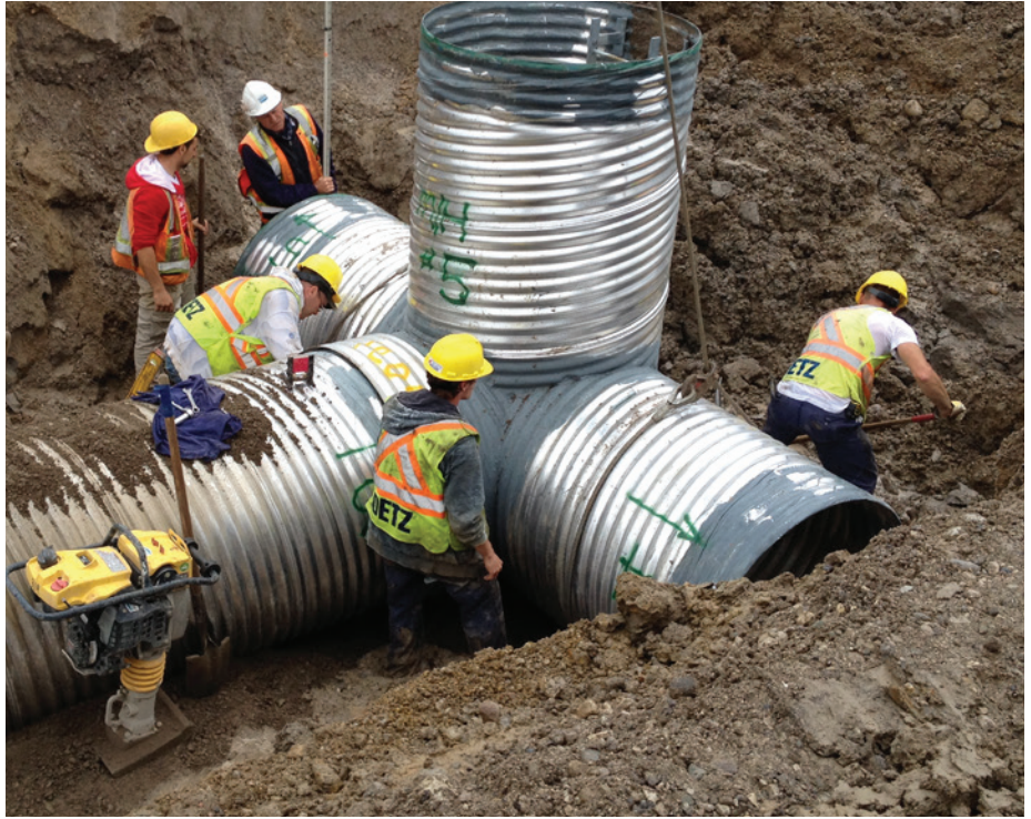
STEECOR'S LIGHTWEIGHT SECTIONS ALLOW INSTALLATION WITHOUT THE NEED FOR HEAVY EQUIPMENT
