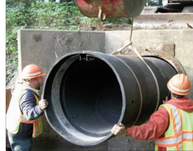
48" CheckMate® Valve replacing a faulty flapgate in a CSO application.
