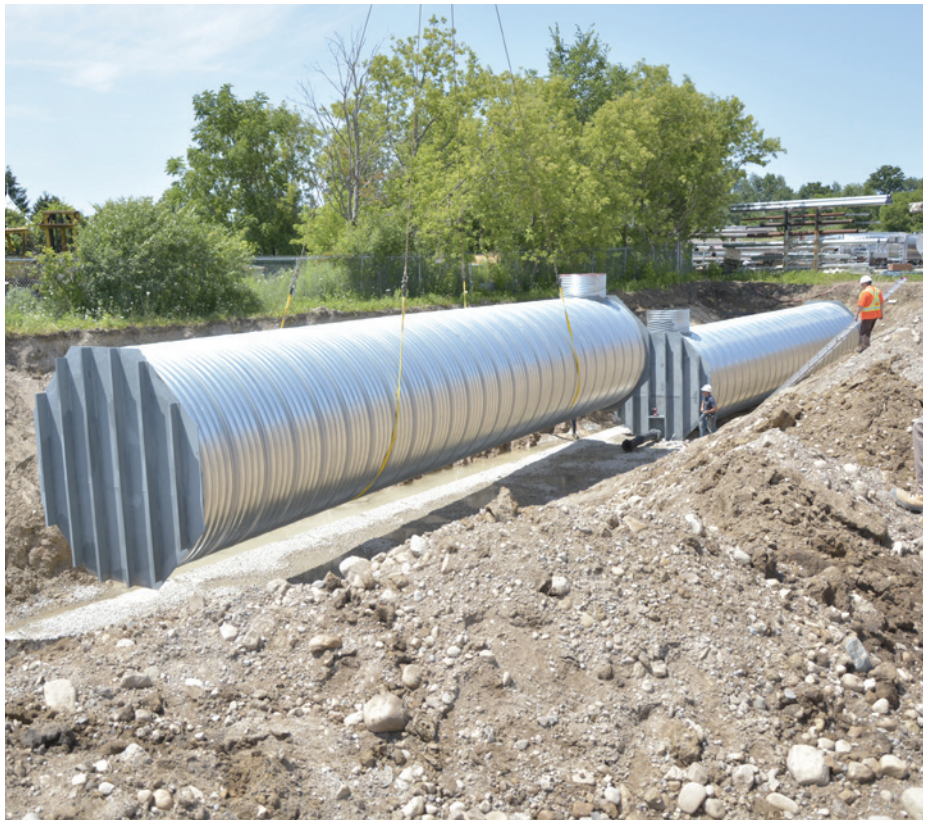
HELICAL CORRUGATIONS AND CONTINUOUS LOCK-SEAM PROVIDE STRENGTH IN A LIGHTWEIGHT STRUCTURE
