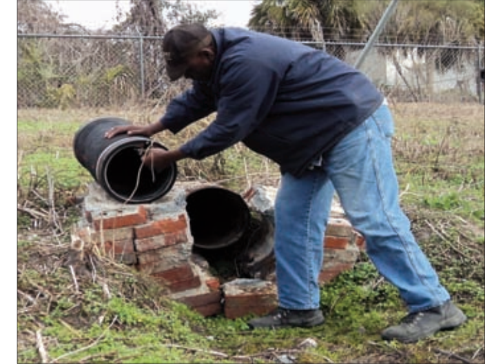
The CheckMate® is also easily installed by hand.
