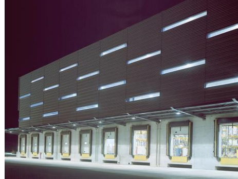
Overhead door facades integrated in the overall building design
