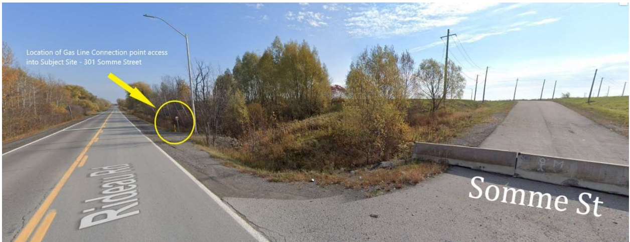
Figure 12: Gas Line Connection Point - (Eastern View corner of Rideau Rd. & Somme St.)
