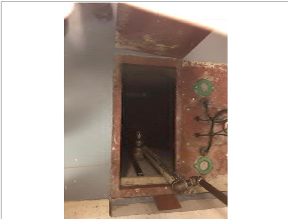
Photograph 16: Example of an elevator sump, dry at the time of the site visit
