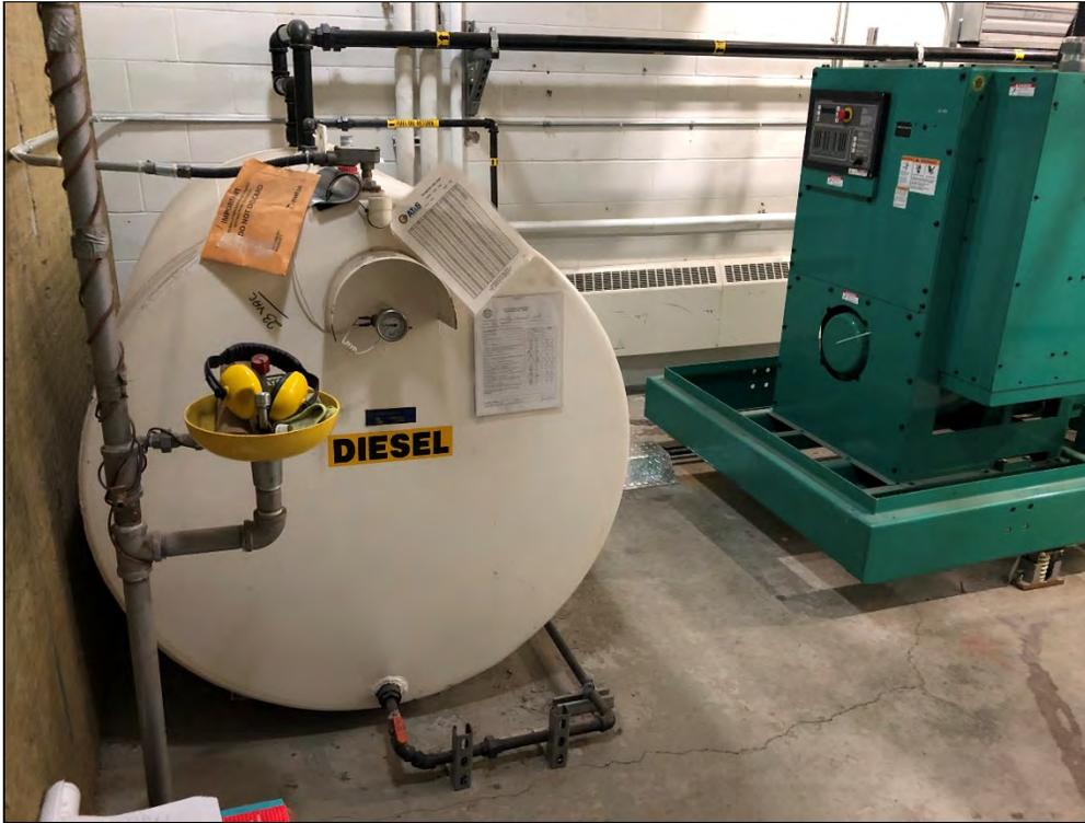
Photograph 7: Diesel AST to fuel backup generator for IT systems
