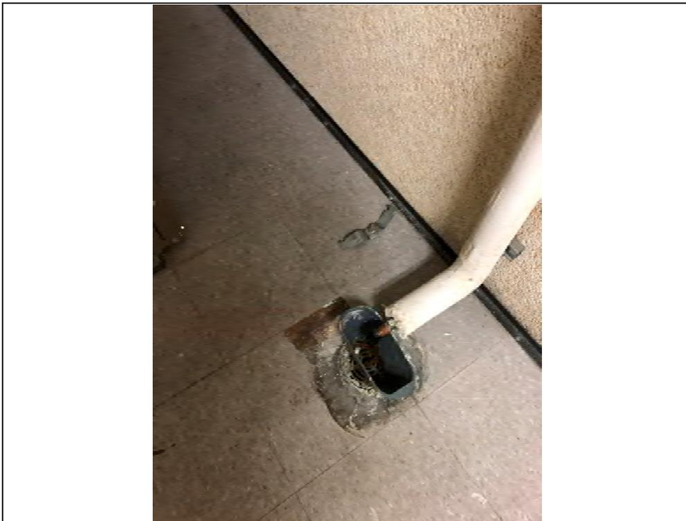
Photograph 14: Example of a drain within the electrical rooms
