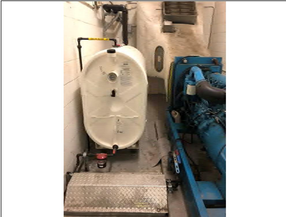
Photograph 8: Diesel AST and backup generator for lighting systems
