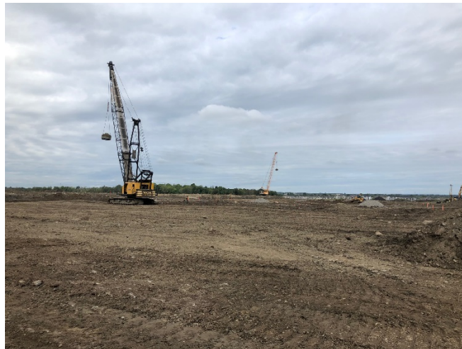
Figure 1. Dynamic Compaction Rig – Ottawa, ON
