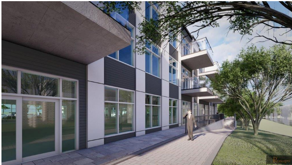
View along Block B facing South
