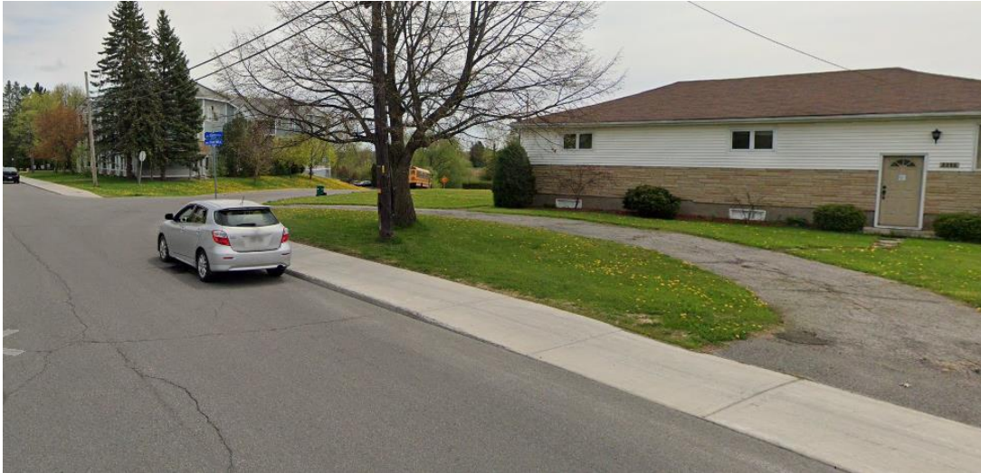
Front of subject property facing East
