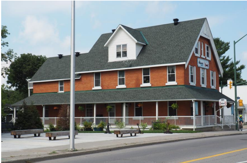
Figure 8: 1510 Stittsville Main Street, formerly known as Green's Hotel. Source: Contentworks, August 2020.
