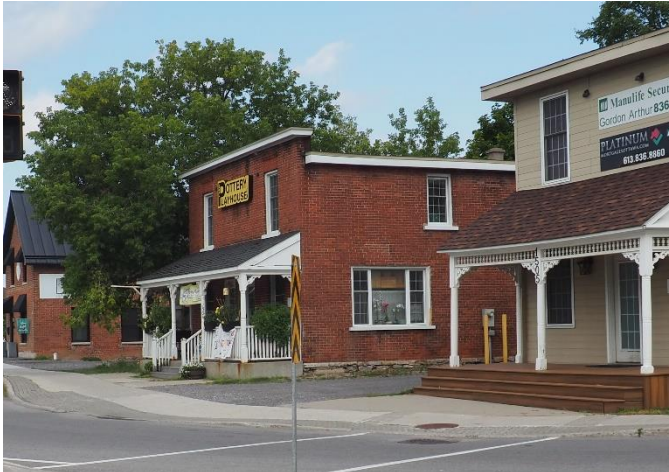
Figure 11: 1501 Stittville Main Street (brick building) located about 90 m from 1518 Stittville Main Street, across the street and on the north side of the former rail line. Source: Contentworks, August 2020.
