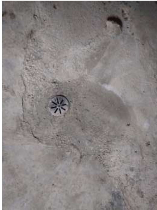
Photograph 9. Floor drain with minor staining, basement 109 Henderson
