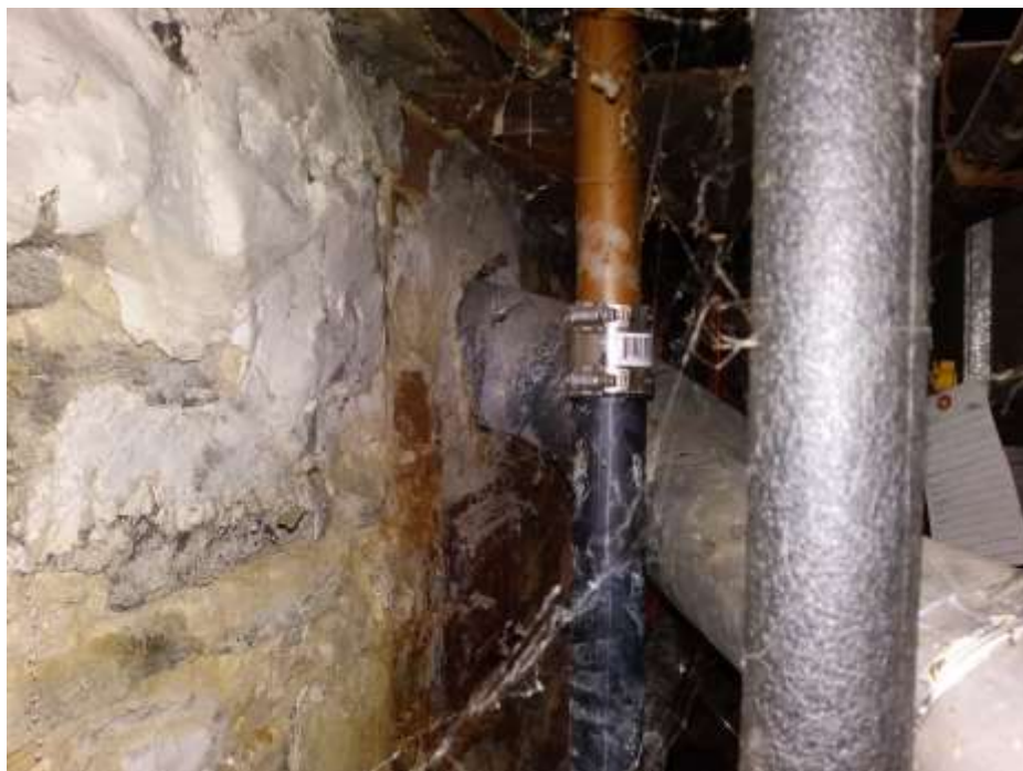
Photograph 11. HVAC ducts and ash clean out port, located behind furnace, basement of 109 Henderson
