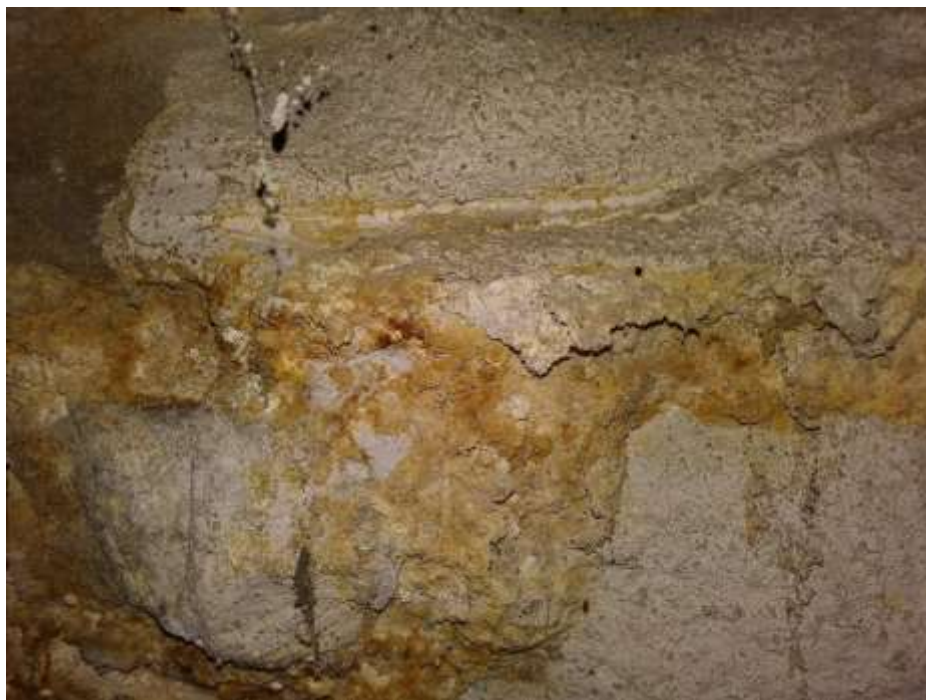
Photograph 12. Unidentified substance (possible efflorescence) on interior of stone foundation, basement of 109 Henderson
