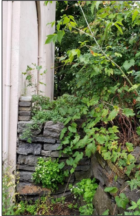
Image 21. View of the south end of the former carriage house, facing northeast. (PR19-032D141)
