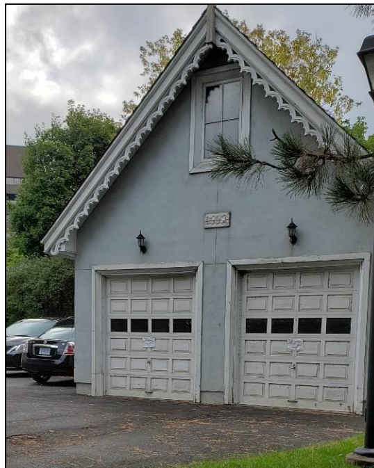
Image 24. View of the garage in the southwest corner of the property, facing south. (PR19-032D129)
