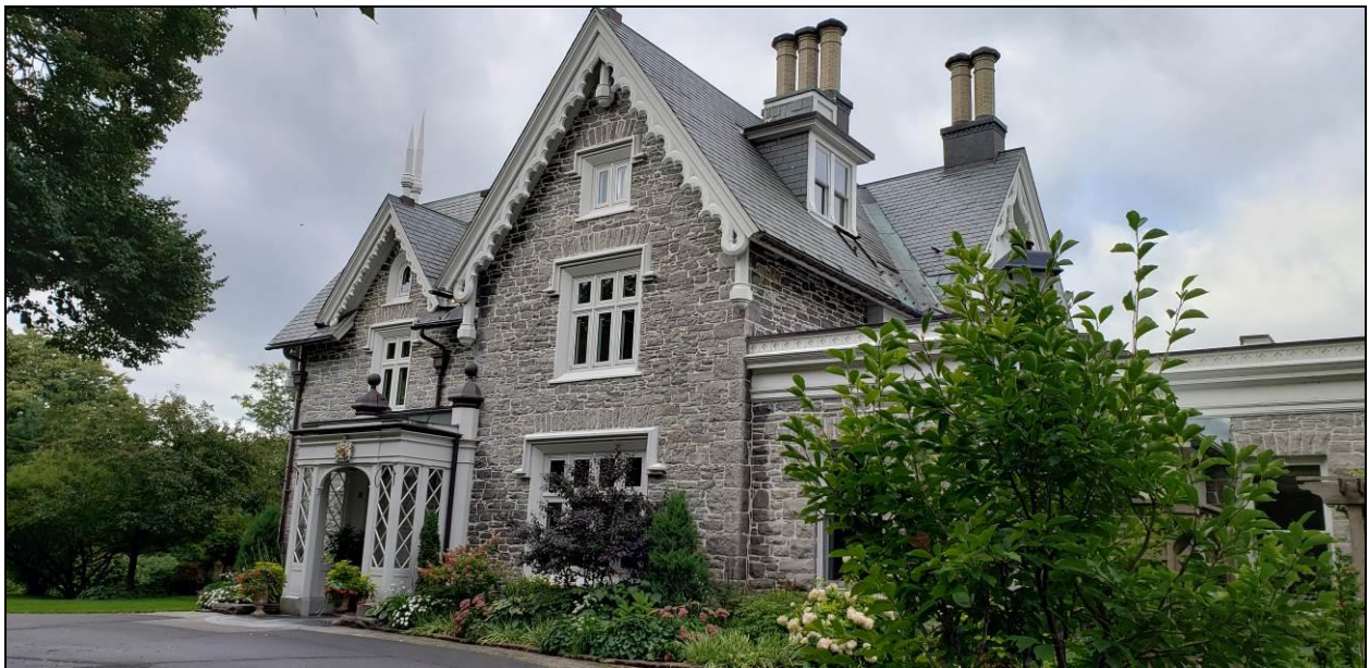
Image 4. View of the east side of Earnscliffe, facing west. (PR19-032D073)
