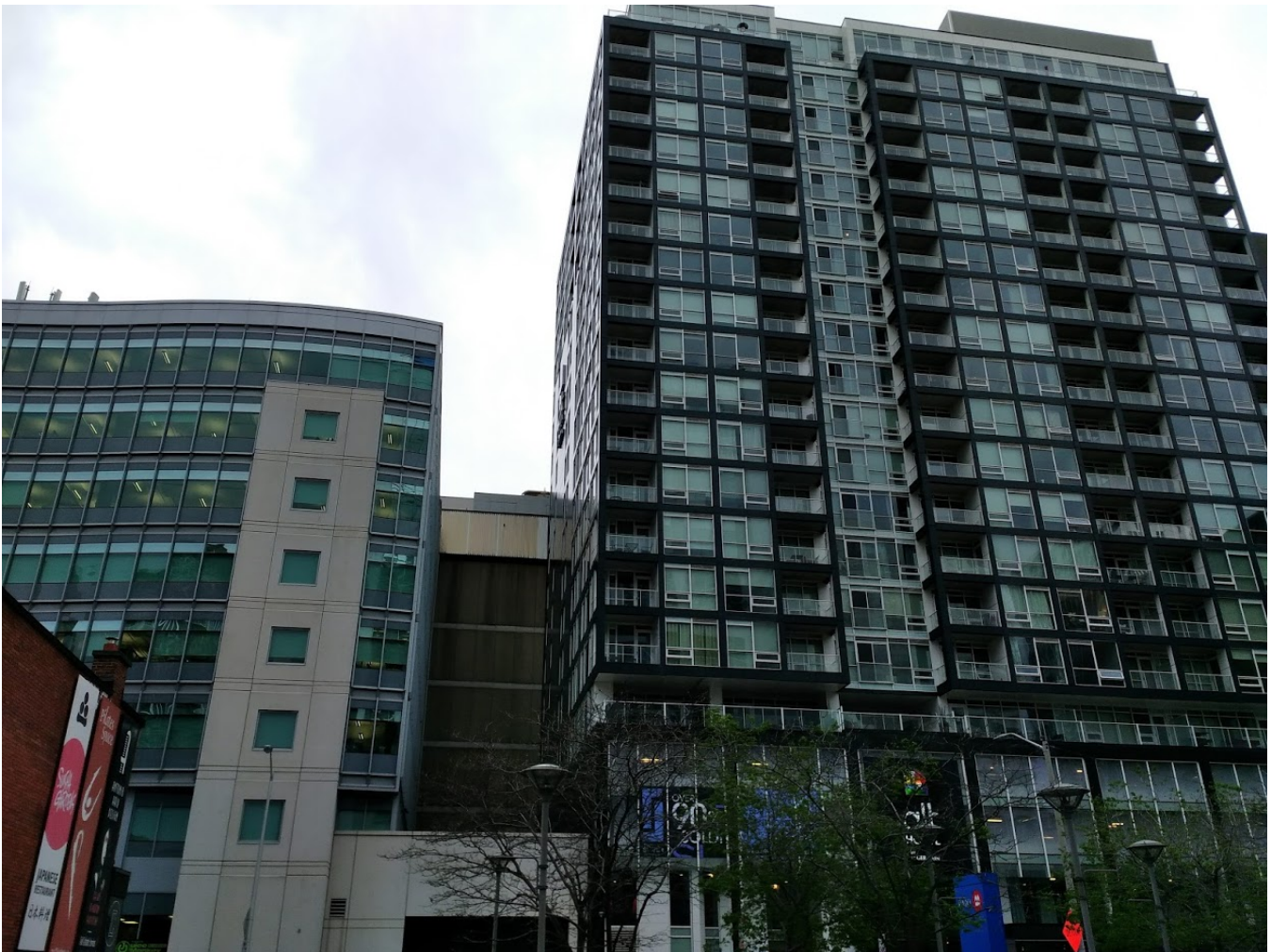
Figure 3: View to the north of the subject property, across Slater Street
