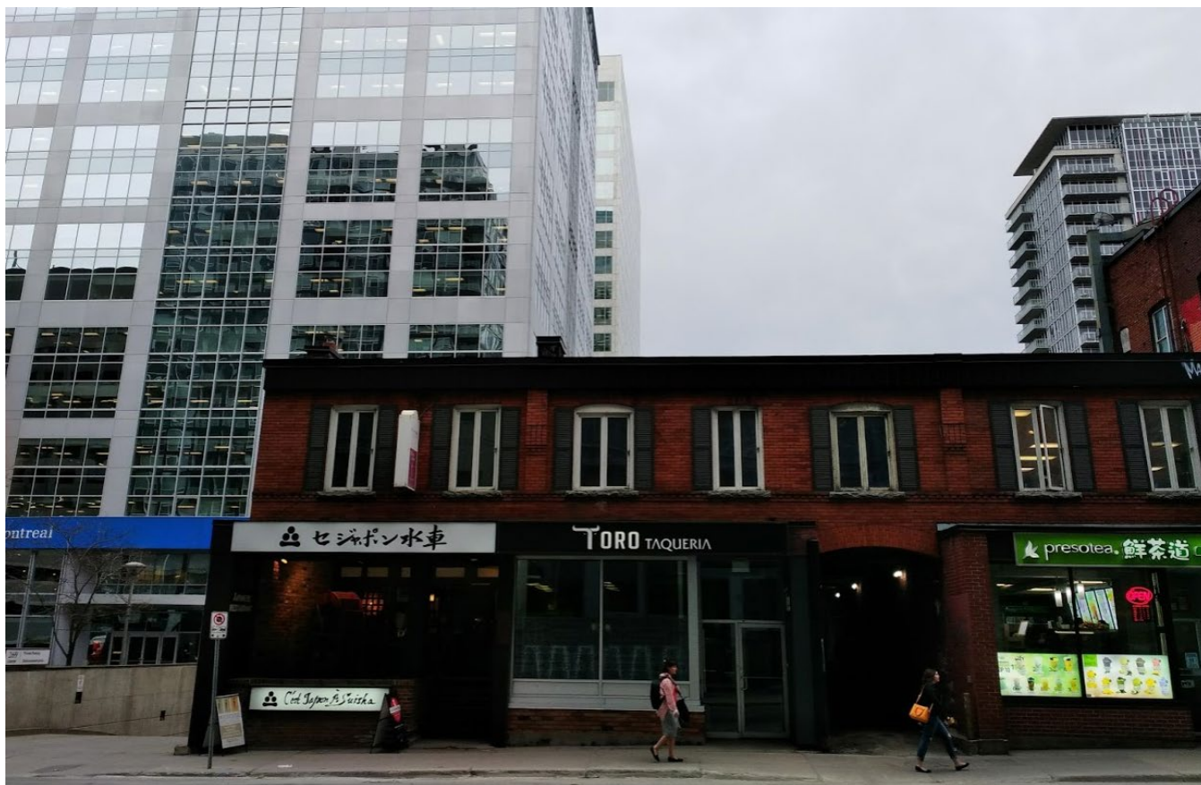
Figure 2: View of the existing two (2) storey building on the subject property from Slater Street
