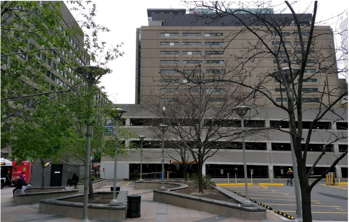
Figure 5: View to the east of the subject property
