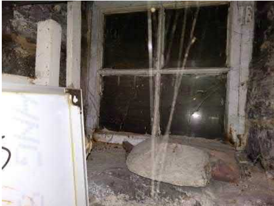
Photograph 5. Windows in basement appear to be buried, basement of 105 Henderson
