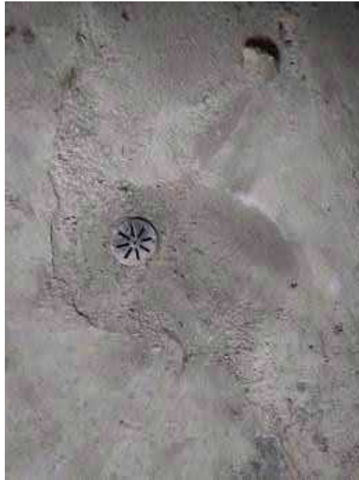
Photograph 9. Floor drain with minor staining, basement 109 Henderson
