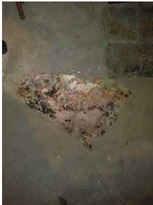
Photograph 9. Floor drain with minor staining, basement 109 Henderson
