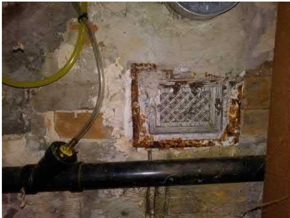
Photograph 5. Windows in basement appear to be buried, basement of 105 Henderson
