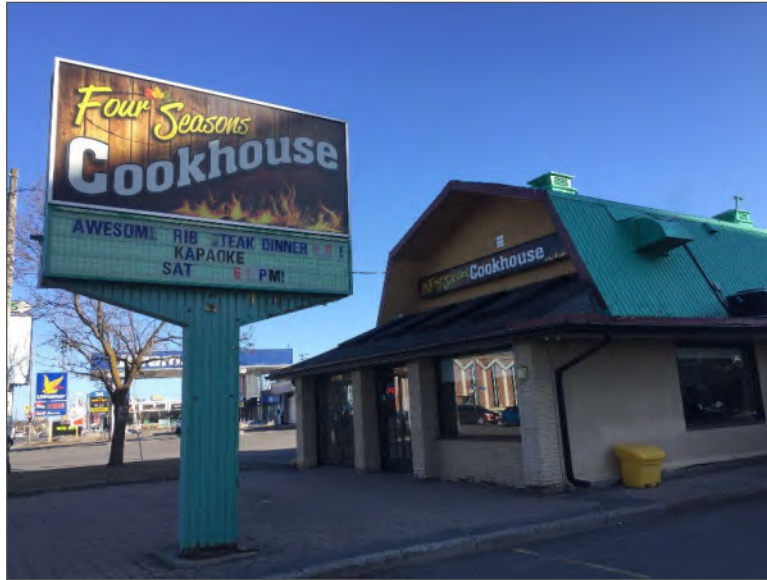
Photo 1 – Site Building (southeast elevation).
