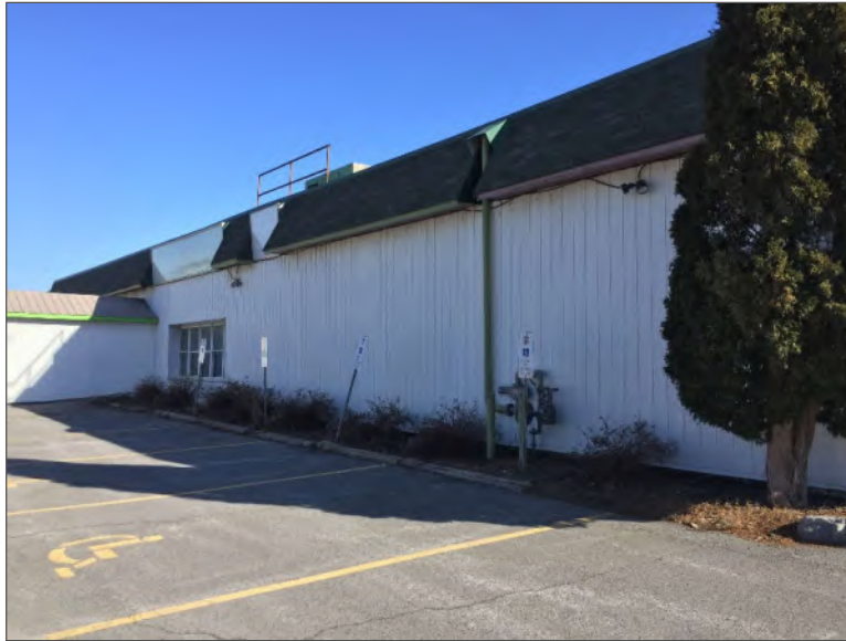
Photo 3 – Site Building B (west elevation).
