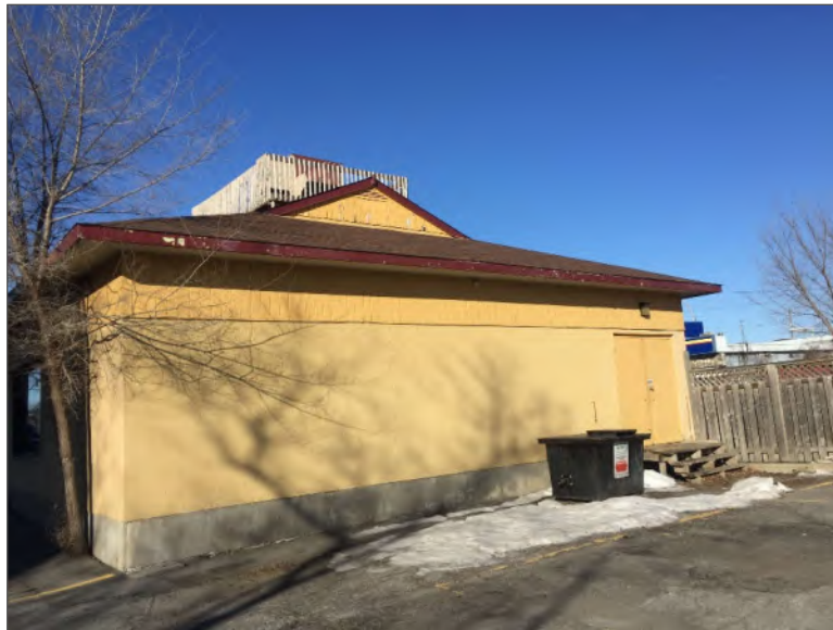
Photo 2 – Site Building A (northeast elevation).
