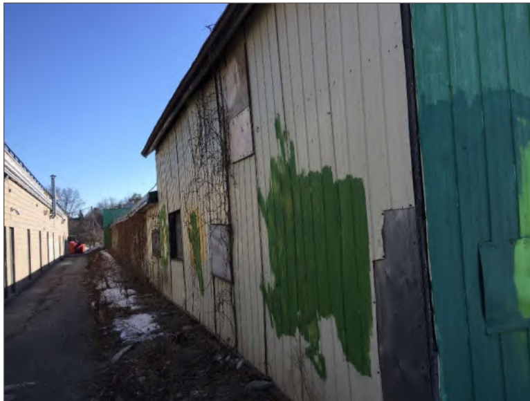
Photo 4 – Site Building (north elevation).
