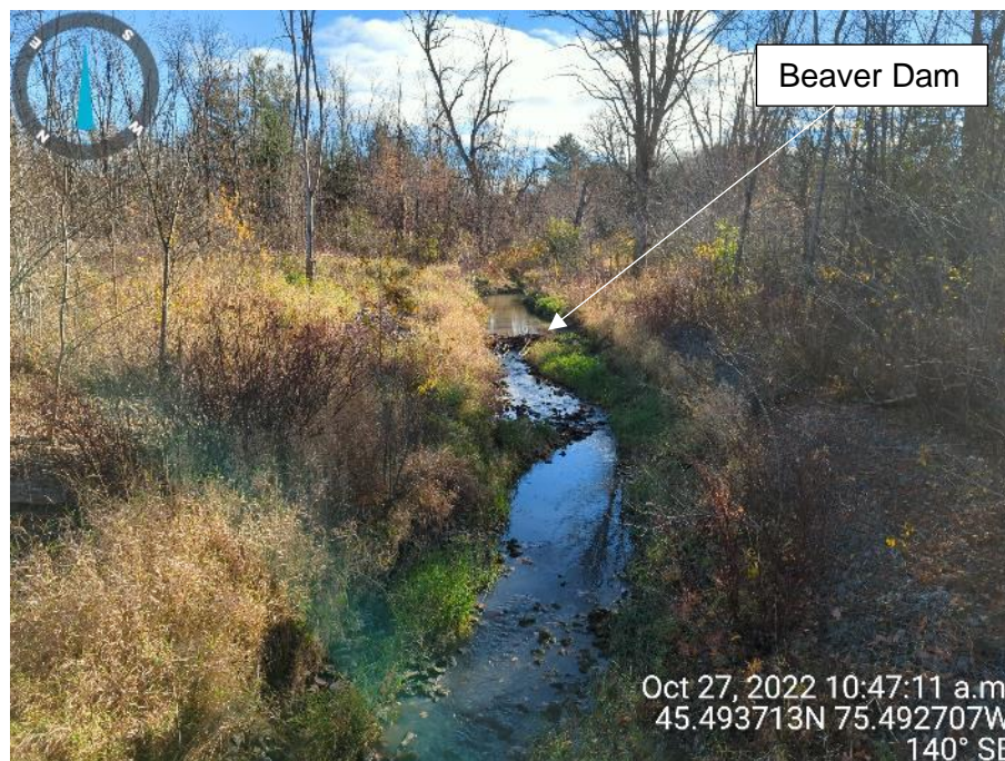
Photo 13: Fish Station looking upstream from the downstream culvert (October 27, 2022)
