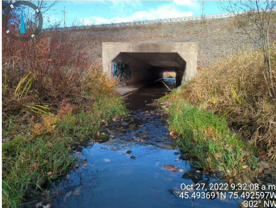
Photo 9: Taylor Creek downstream end, looking downstream at the culvert flowing under Jeanne d'Arc Boulevard North (October 27, 2022)
