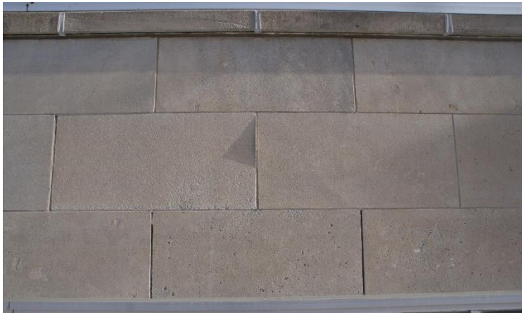
Figures 7: View of the Niagara limestone cladding above the Kent Street entrance. Note the variations in the material, coursing and the window sill course band the length of units corresponding with the cladding coursing. Mortar is missing from a number of joints. Source: Commonwealth 2023.
