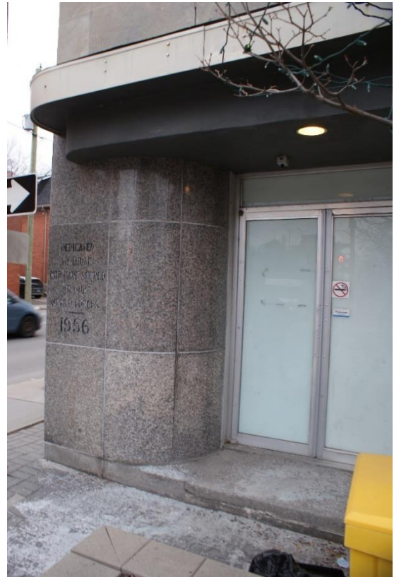
Figures 19 & 20: Detail section of the Gilmour Street Entrance illustrating the form and materials and the relationship to the entrance doors. Existing view of the canopy illustrating alterations to the canopy and entrance doors. Source: Original 1955 Drawing Set A5 & Commonwealth 2022.
