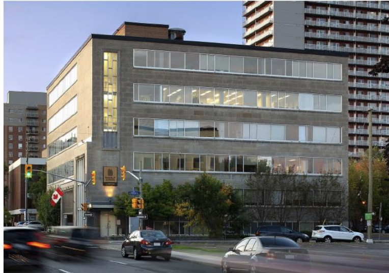
Figure 2 - Current condition, 2022, of Legion House
