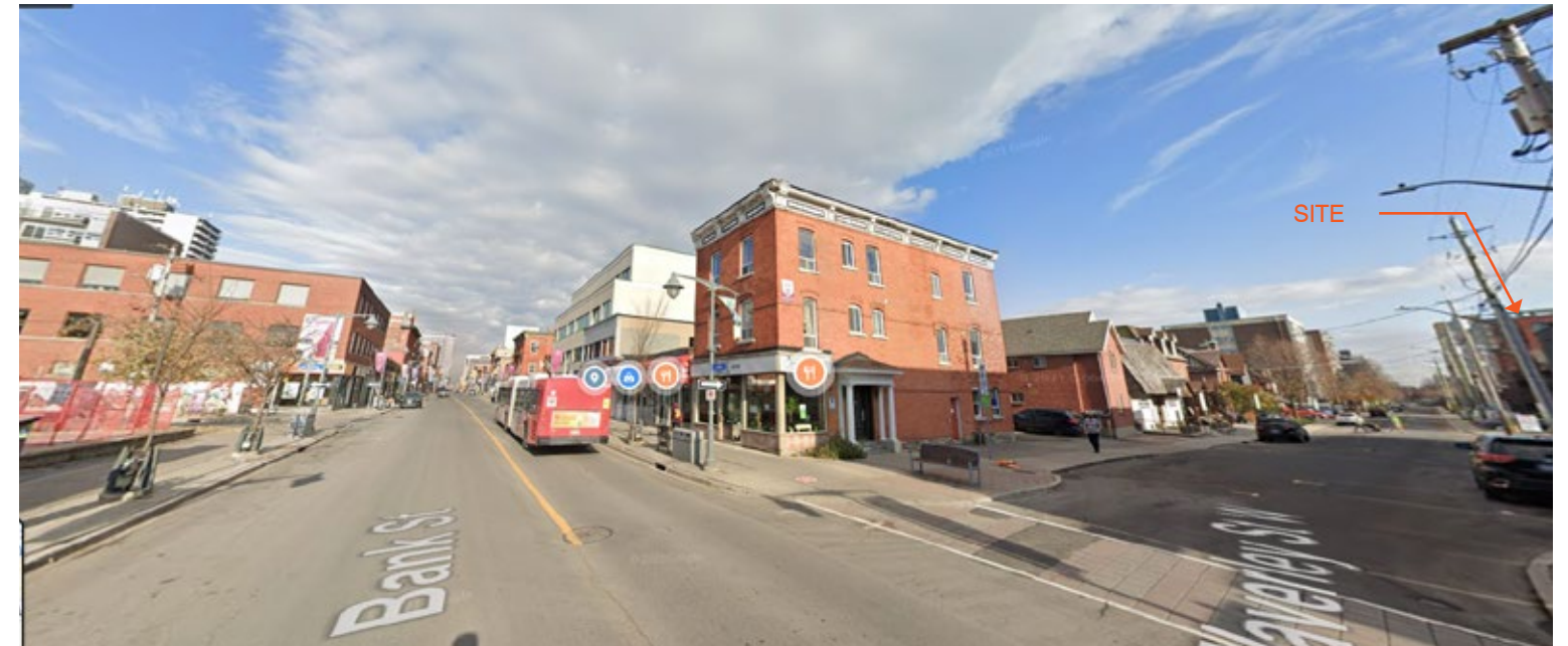
8 - VIEW FROM BANK ST / WAVERLEY ST LOOKING NORTH-WEST
