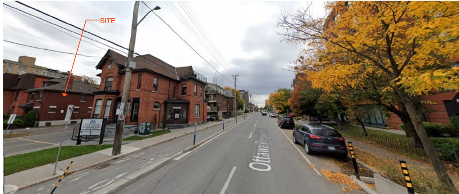
5 - VIEW FROM WAVERLEY ST. / O'CONNOR ST. LOOKING SOUTH-EAST
