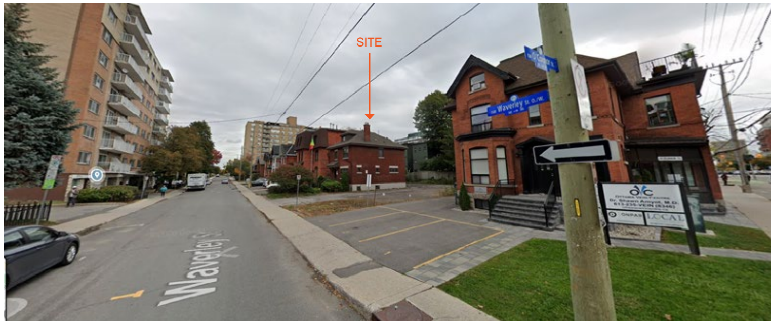
3 - VIEW FROM WAVERLEY ST./O'CONNOR ST. LOOKING EAST AT SITE
