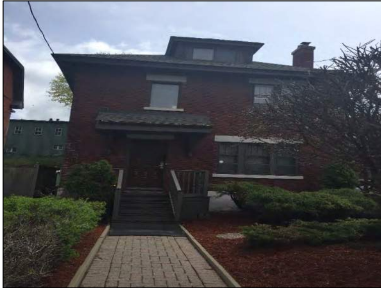
Photo 1 – Site Building (north elevation).
