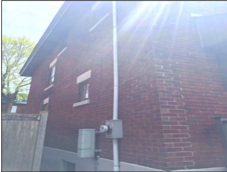
Photo 3 – Site Building (east elevation).
