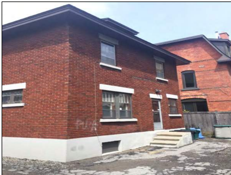
Photo 2 – Site Building (south elevation).
