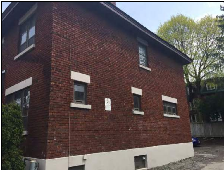
Photo 4 – Site Building (west elevation).
