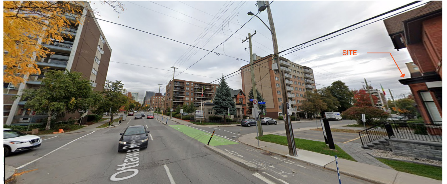
6 - VIEW FROM O'CONNOR ST. LOOKING NORTH-WEST
