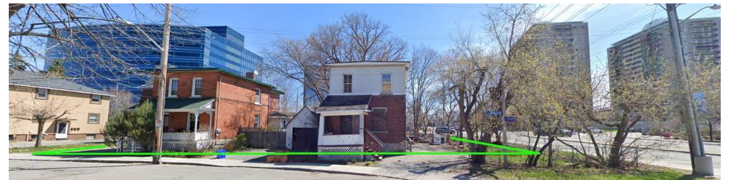
Gardner frontage of subject property
